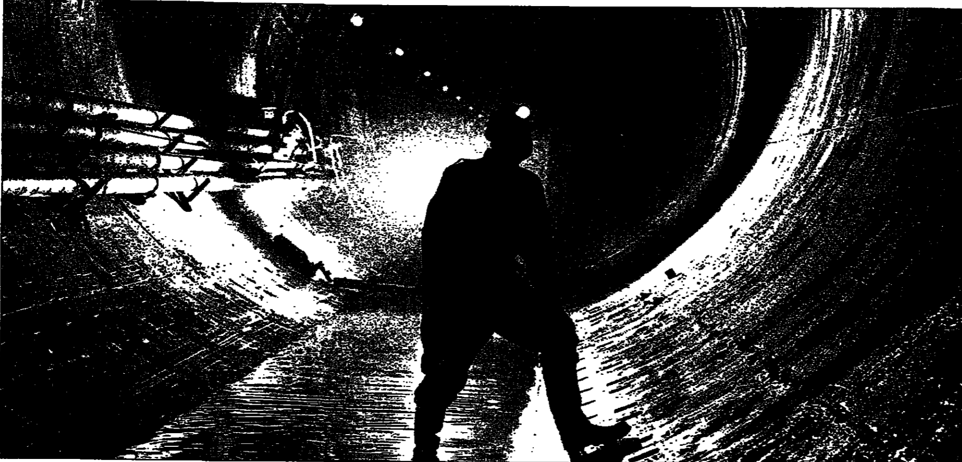
Mike Kinski, new Southern Water chief executive, inspects the three-mile stormwater tunnel which will prevent sewage overflow onto Brighton beach. PHOTOGRAPH: ROGER SAMBER
